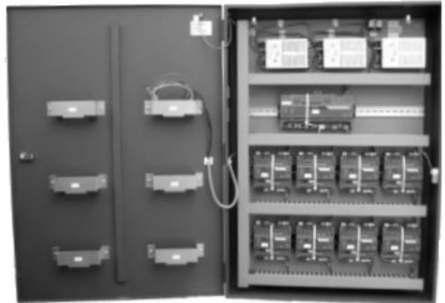
Figure 1: Security Control Panel Mounted in a 30 in. x 42 in. Enclosure
